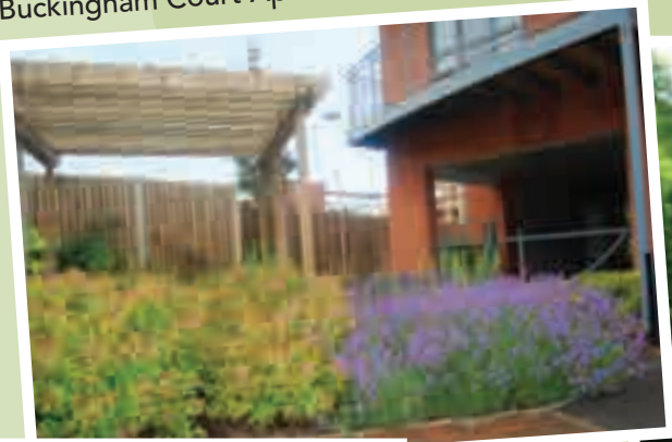
Buckingham Court Apartments
