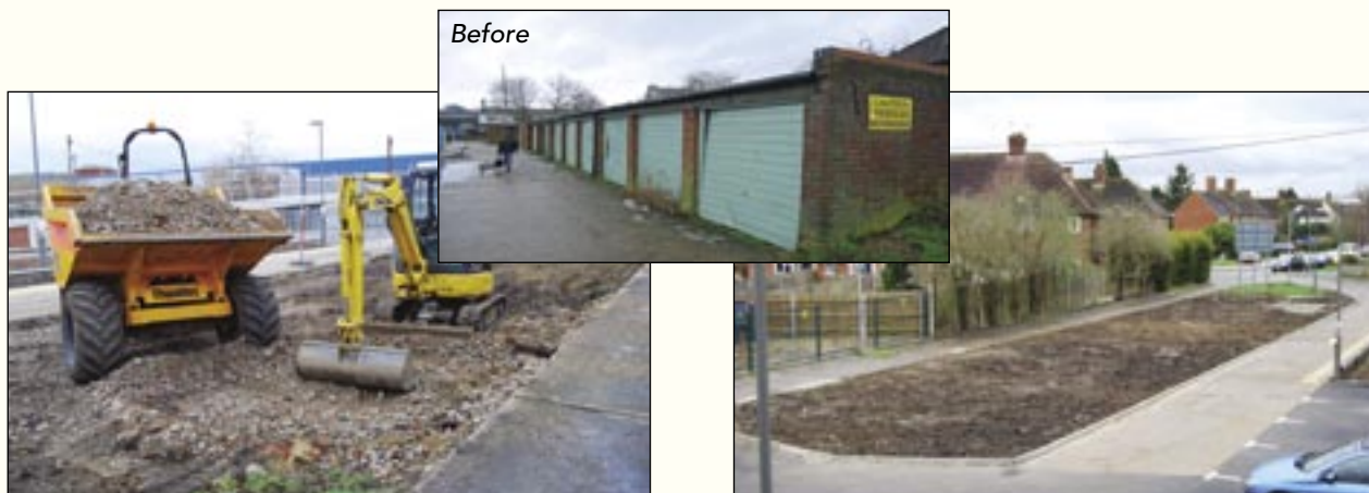
Clearing the concrete. Photo by K. Turner
