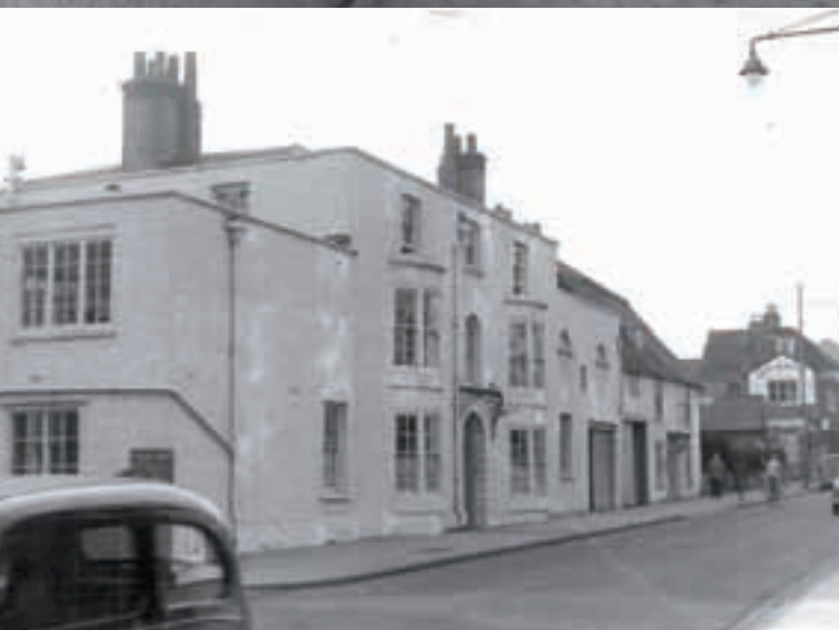
Walton Street in 1956 showing the buildings that were demolished to make way for the County Tower.
