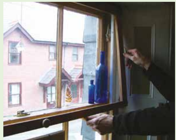
Hinged secondary glazing - bar aligned with original windows for a good match. Photo courtesy of www.superhomes.org.uk
