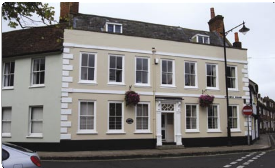
Temple House after being renovated Photo taken by Keith Turner
